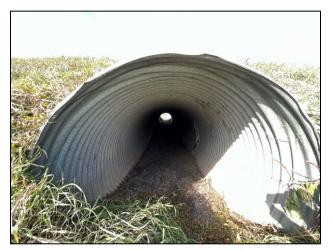
The third culvert is located approximately 143 feet west of Iowa Ave and just under where the end of the asphalt section of the road. This is a 60" CMP x 50' long installed in 1978. The pipe had a slight "egg" shape to it with a slight amount of sediment on the bottom. It was also observed a bore machine had punctured the southeast side of the culvert in 2 different spots. Cover over the pipe was greater than 48" at the shoulder.
