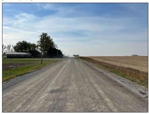
**Drainage**: Ditches are graded at a 2H:1V (H=horizontal, V=vertical) foreslope with a ditch bottom depth of about 48"-54". There are 3 culverts that cross the roadway north and south.
